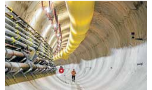
First section of the Metro Tunnel complete
