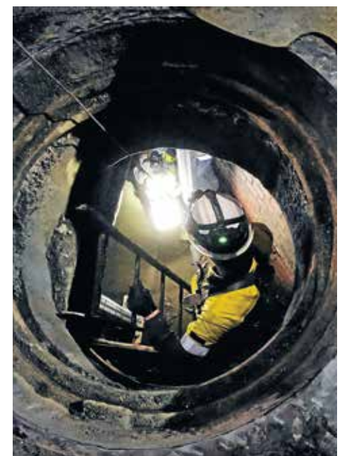
▲ A worker inspects a CBD pit.
