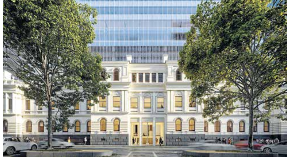
▲ A render of the front of the building.
