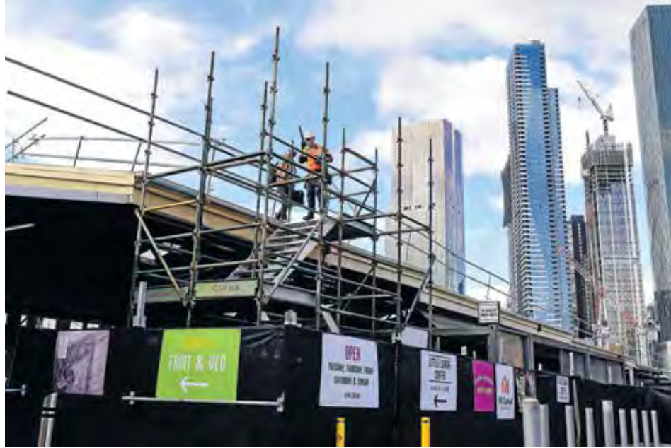
▲ Work continues on restoring the Queen Victoria Market's heritage sheds.
