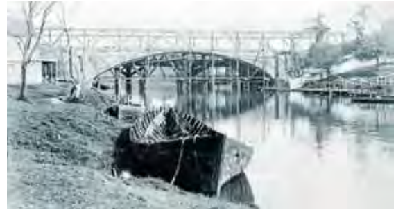
▲ Princes Bridge during demolition 1885. RHSV_PH-100109.
