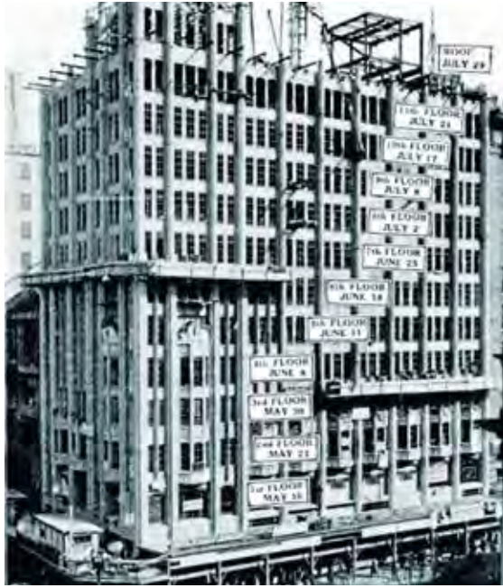
▲ Construction of Manchester Unity, 1932. RHSV BL011-019.002.
